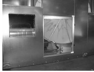
FIGURE 26: Access to wheel through exhaust blower door.
